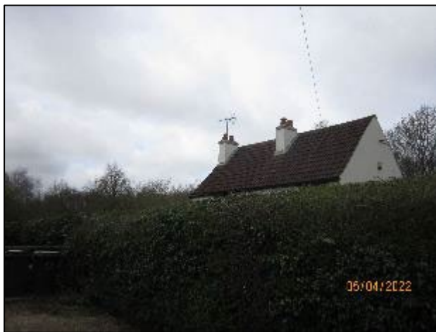
Photograph showing adjacent neighbouring property 145 Moorgreen, located north of the application site.
